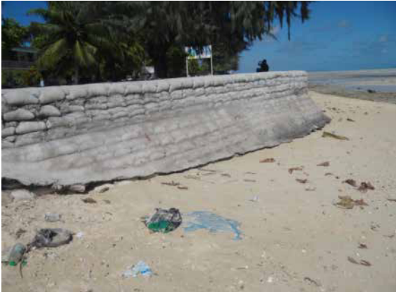
Photo 7: Grout-filled sandbags (Credit: Shand 2015)
