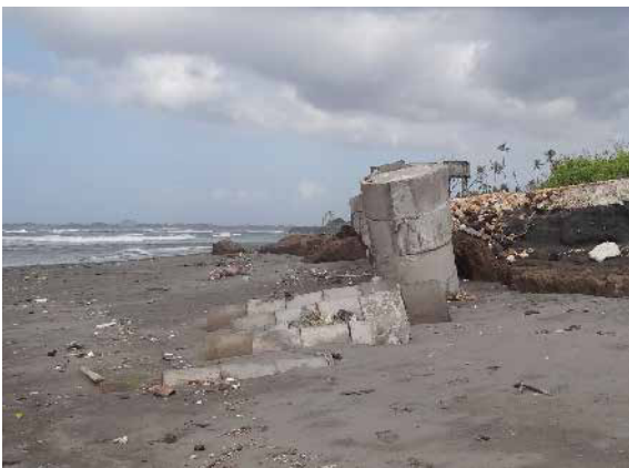
Photo 11: Concrete filled drums
