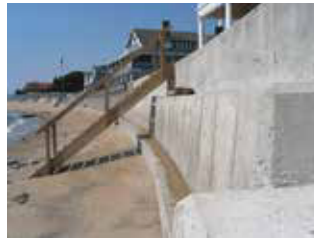
Example stepped seawall (Coastline consulting LLC)
