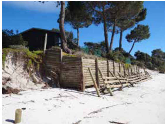
Timber pile retaining wall in New Zealand being undermined and outflanked (source: Shand, 2014)
