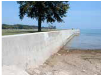
Example of vertical seawall at Lake Erie (ohiodnr.gov)
