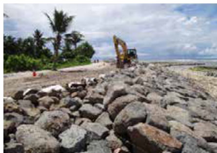
Photo 2: Rock revetments (Shand) in Kiribati
