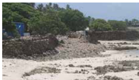
Photo 4: Stacked coral block wall in Kiribati collapses forming a 'dynamically stable revetment' (Credit: Shand)
