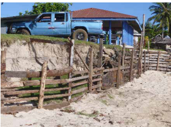
Photo 13: Rock filled timber wall
