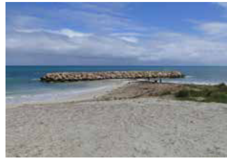
Photo 5 and Photo 6: Beach Tombolo created in lee of an offshore breakwater in Geraldton, Western Australia (Credit: Shand)
