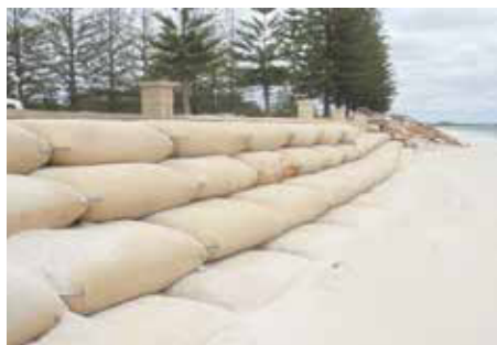
Photo 1: Semi-rigid geotextile container (Maccaferri NZ Ltd.)
